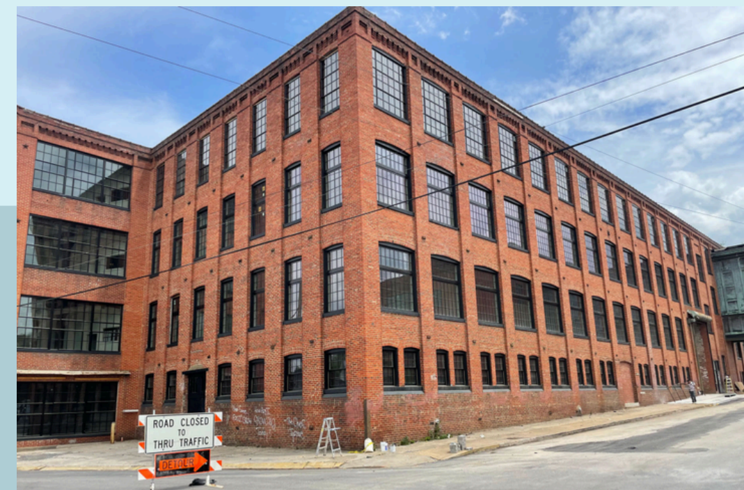
Interwoven Mills Buildings 1-6, Martinsburg
