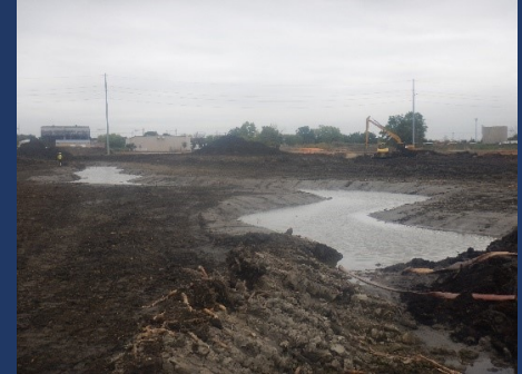
South Wilmington Wetlands Park Construction (City of Wilmington, DE Website)
