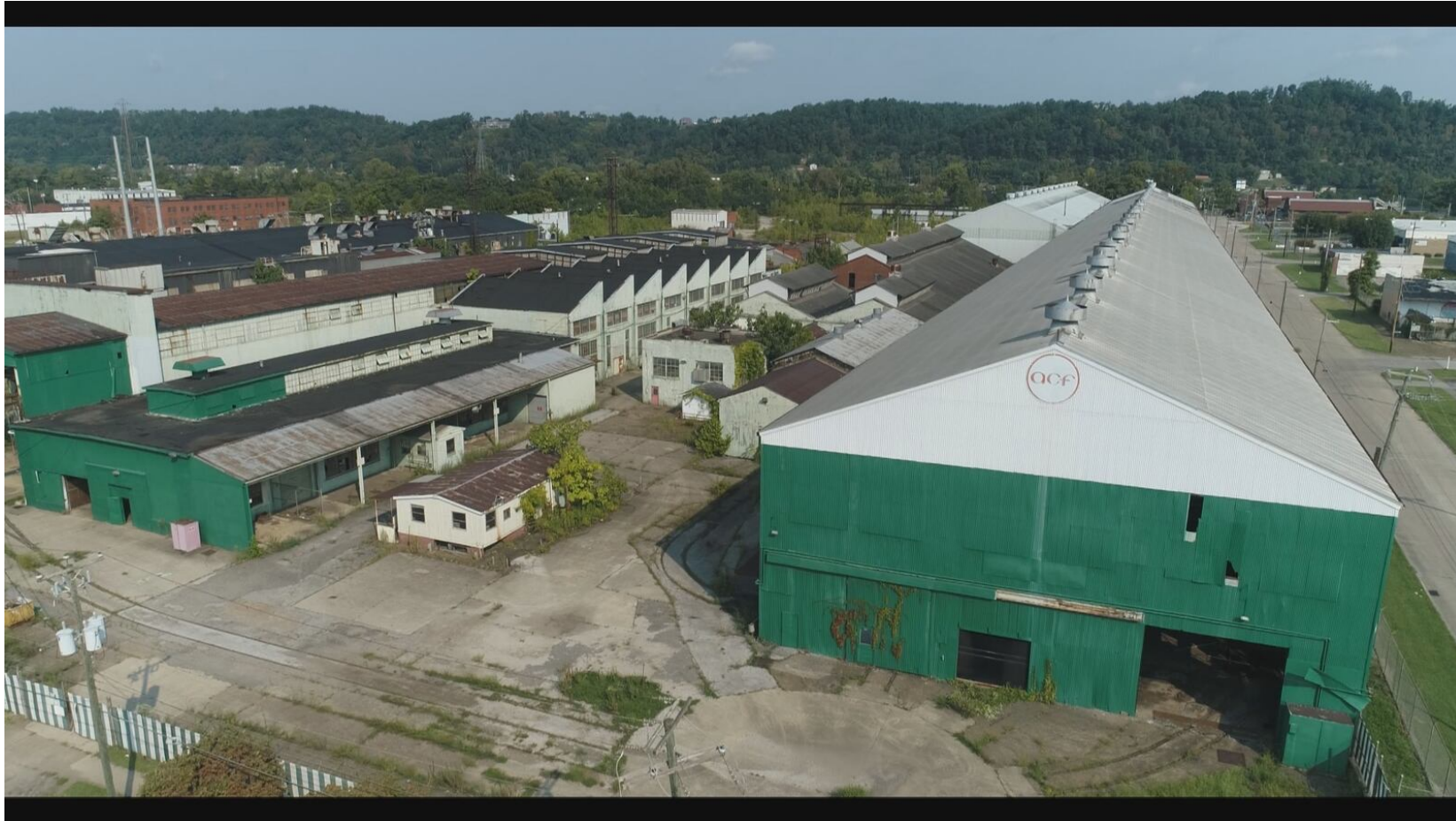
American Car Foundry Site (Huntington, WV) The plant manufactured railcars and rail car parts from the 1880s to 2010.
