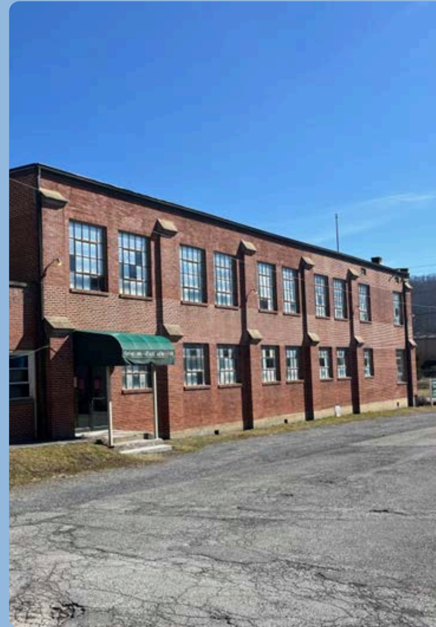
Marshall University Former Clifford Armory
